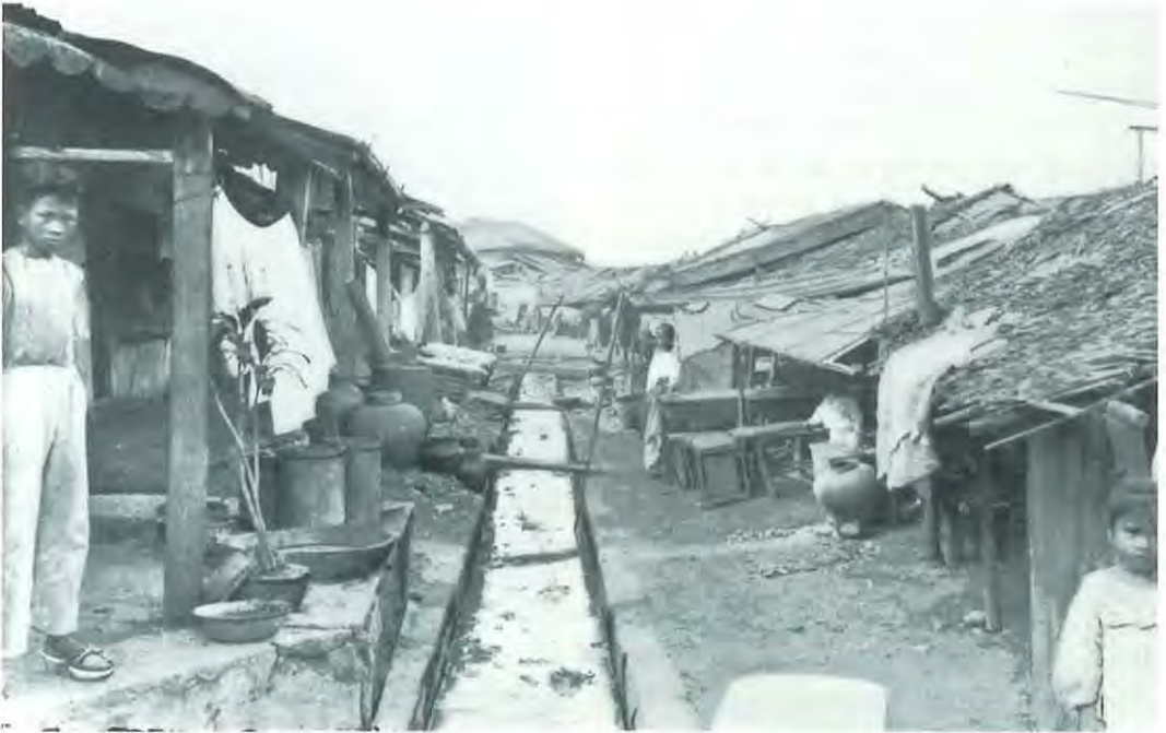
A SEWAGE-CLOGGED DRAINAGE DITCH, used by Filipino vendors and families
